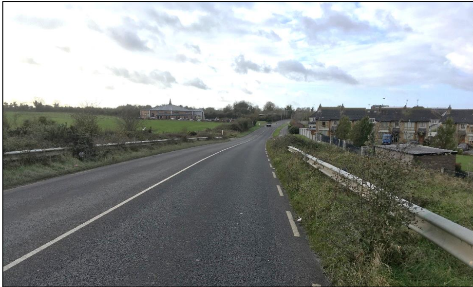
Figure 2.4: Colpe Road Carriageway (Source: google.ie)
